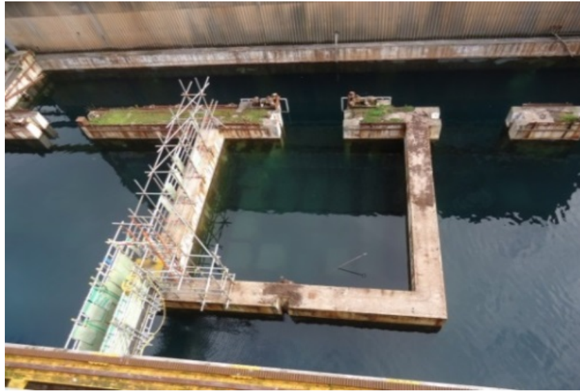
Fig. 7. Pond Walls After
