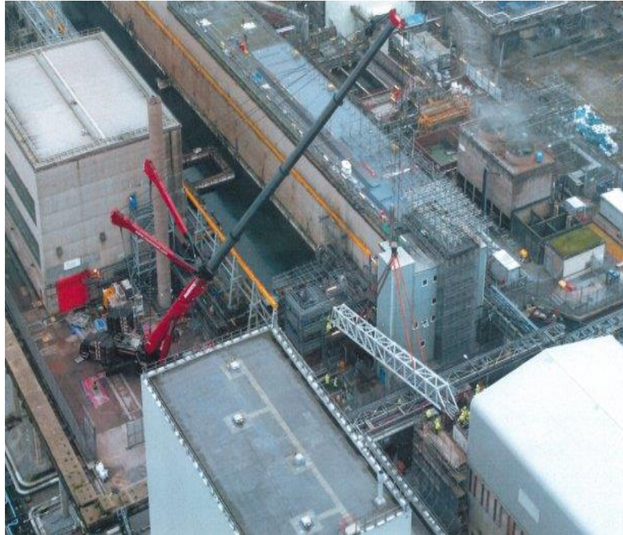
Fig. 5. Pipe Bridge Installation
