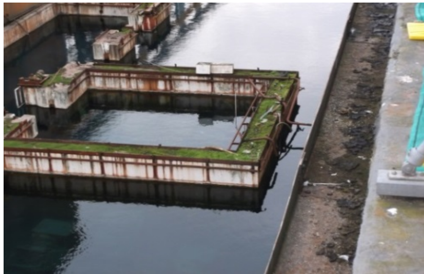
Fig. 6. Pond Walls Before
